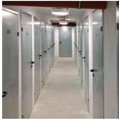
RESIDENTIAL ESTATE UNIVERSAL DOORS TO UTILITY ROOMS
